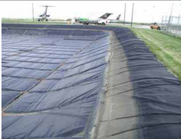
Birds are permanently excluded from this storm water detention facility through the use of a floating permeable barrier (Photo courtesy Industrial & Environmental Concepts, Inc.).
