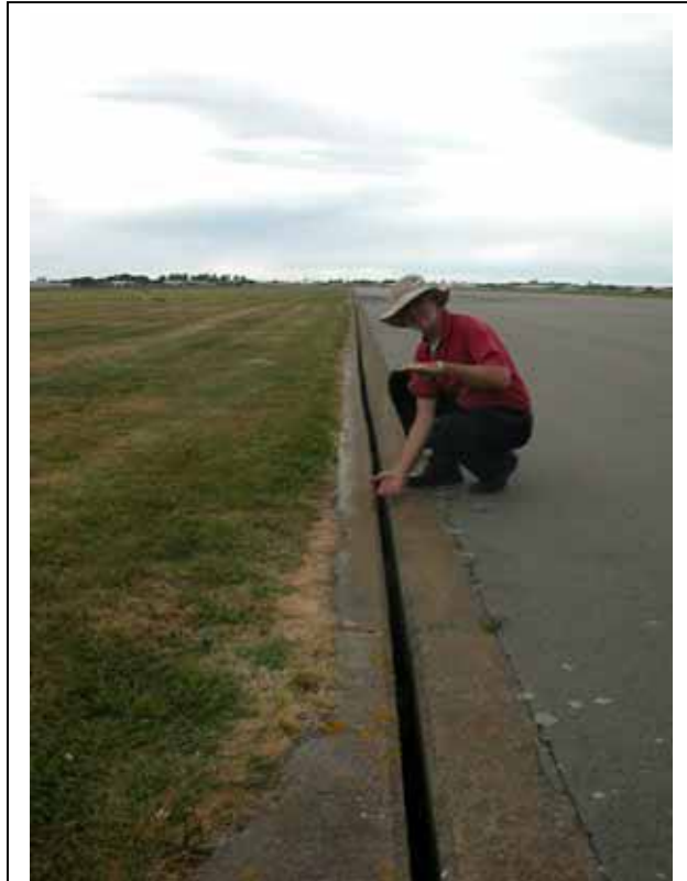
Earthworms crawling onto runways after heavy rains can be a strong attractant to gulls and other birds. This runway in New Zealand uses slit drains to block worms from reaching the runway. Other options include brush-sweeping runway edges to remove worms and deploying extra personnel to disperse gulls. As of 2005, there are no chemicals registered in the USA to control earthworms (photo by R. A. Dolbeer, USDA).
