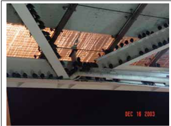
Elimination of wildlife habitat and attractants on or near airports will reduce wildlife strikes. Exposed I beams, such as used in the canopy over the passenger pick-up area at a Midwestern USA airport, make ideal roosting habitat for flocks of European starlings (photo by R. White, USDA).
