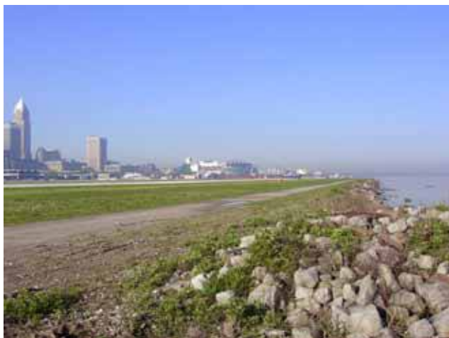
During the first winter following its completion, over 20,000 Bonaparte's gulls used this dredge spoil containment area (far right of photo) constructed next to an airport on Lake Erie's shoreline. The airport's main runway can be seen to the left (photo by E. Cleary, FAA).
