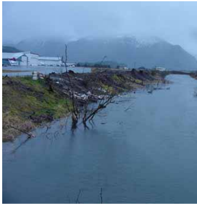
Bodies of open water adjacent to airports, such as this drainage canal, are often magnets for waterfowl and wading birds. Note the shallow slope that allows birds easy access in and out of the water. Such canals should be covered if possible or diverted away from the airport (photo by E. Cleary, FAA).
