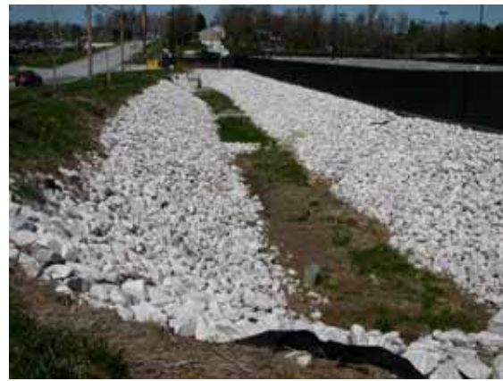
Water detention basins at airports, such as this French-drain system at an eastern USA airport, should be designed to completely drain within 48 hours after the design storm event (photo by R. A. Dolbeer, USDA).
