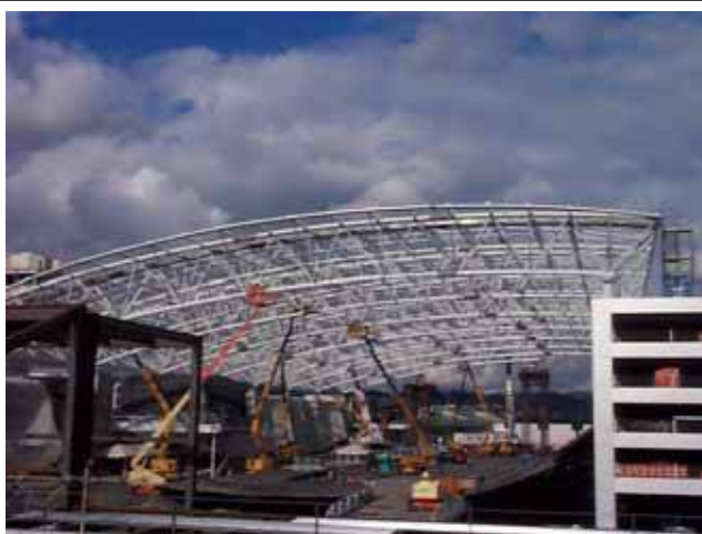
Within 2 weeks of completion, starlings and pigeons had started roosting in this canopy constructed over the passenger drop-off area at a major USA airport (photo by S. Gordon).
